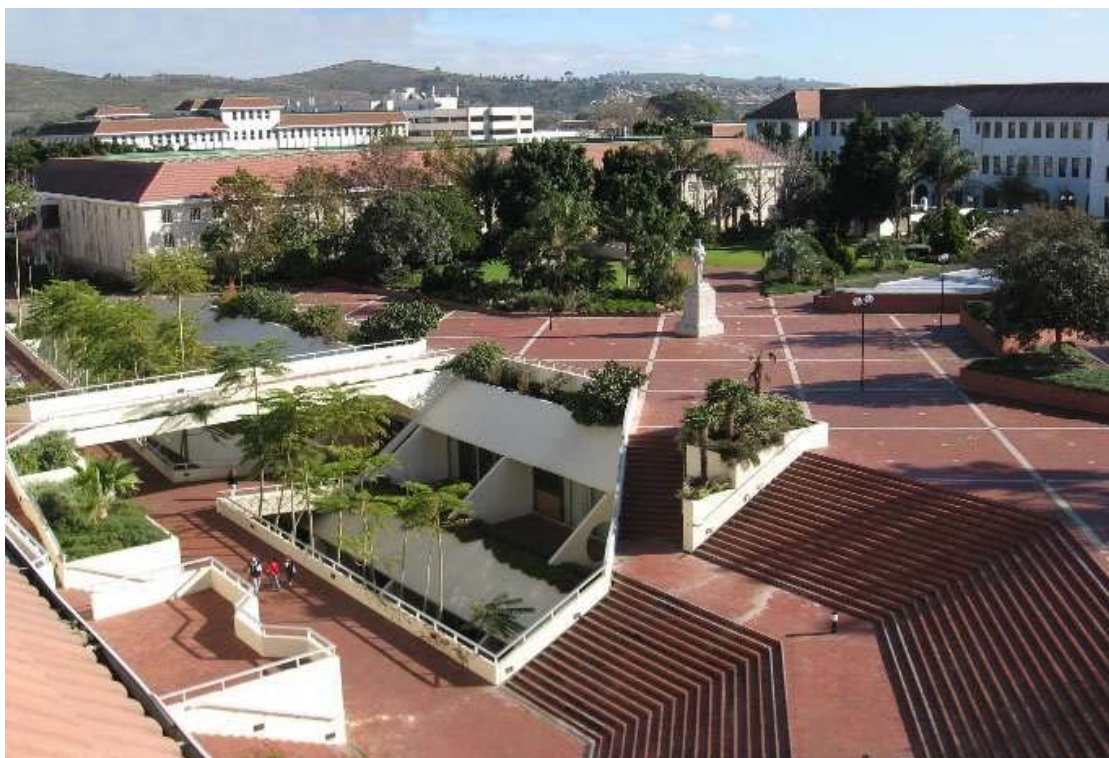
The JS Gericke Library of Stellenbosch University, built under the central Jan Marais Square so as not to mar the aesthetics of the historic buildings on the site.
