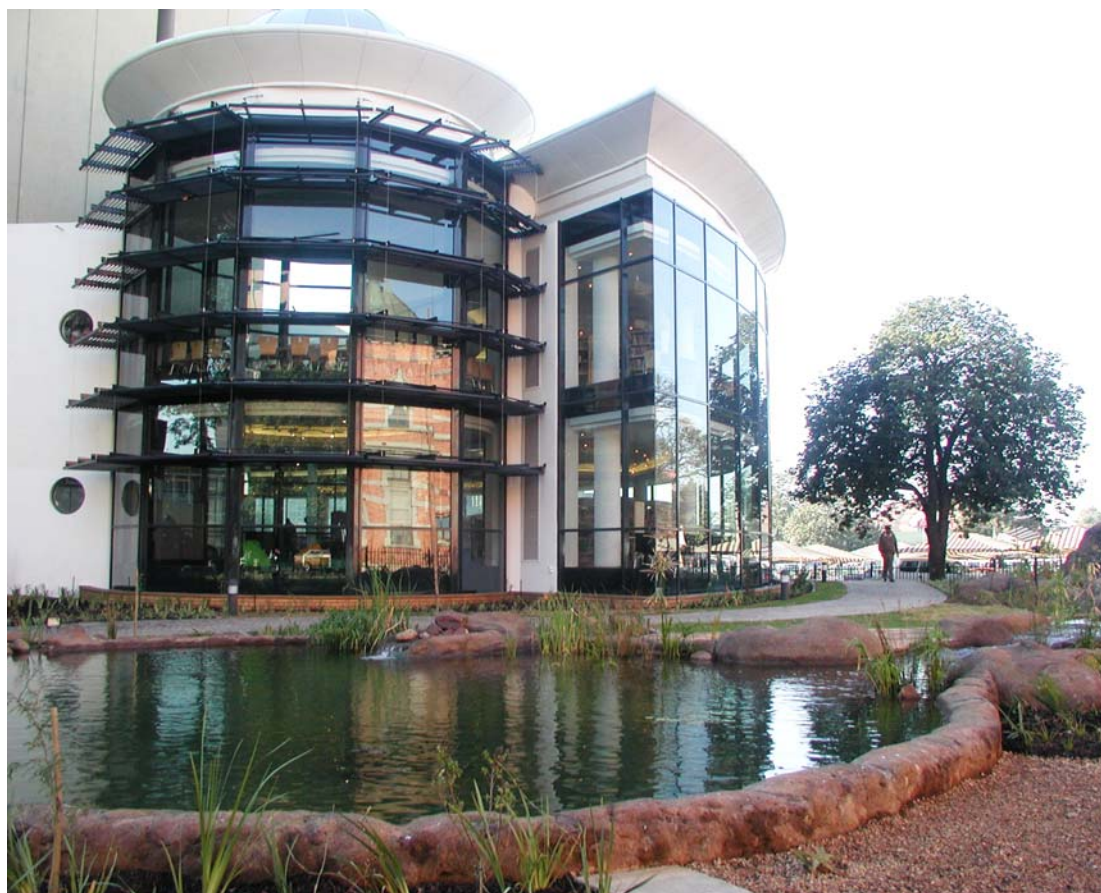
The distinctive architecture of the glass-fronted Msunduzi Municipal Library in Pietermaritzburg, sponsored in part by the Carnegie Corporation of New York.
