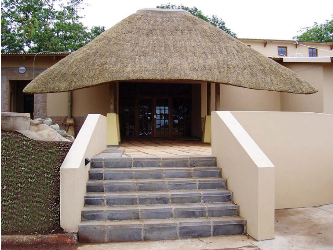
The new 500 square metre Nongoma Library in rural KwaZulu-Natal, which opened in 2006, was for many years housed in a single room.
