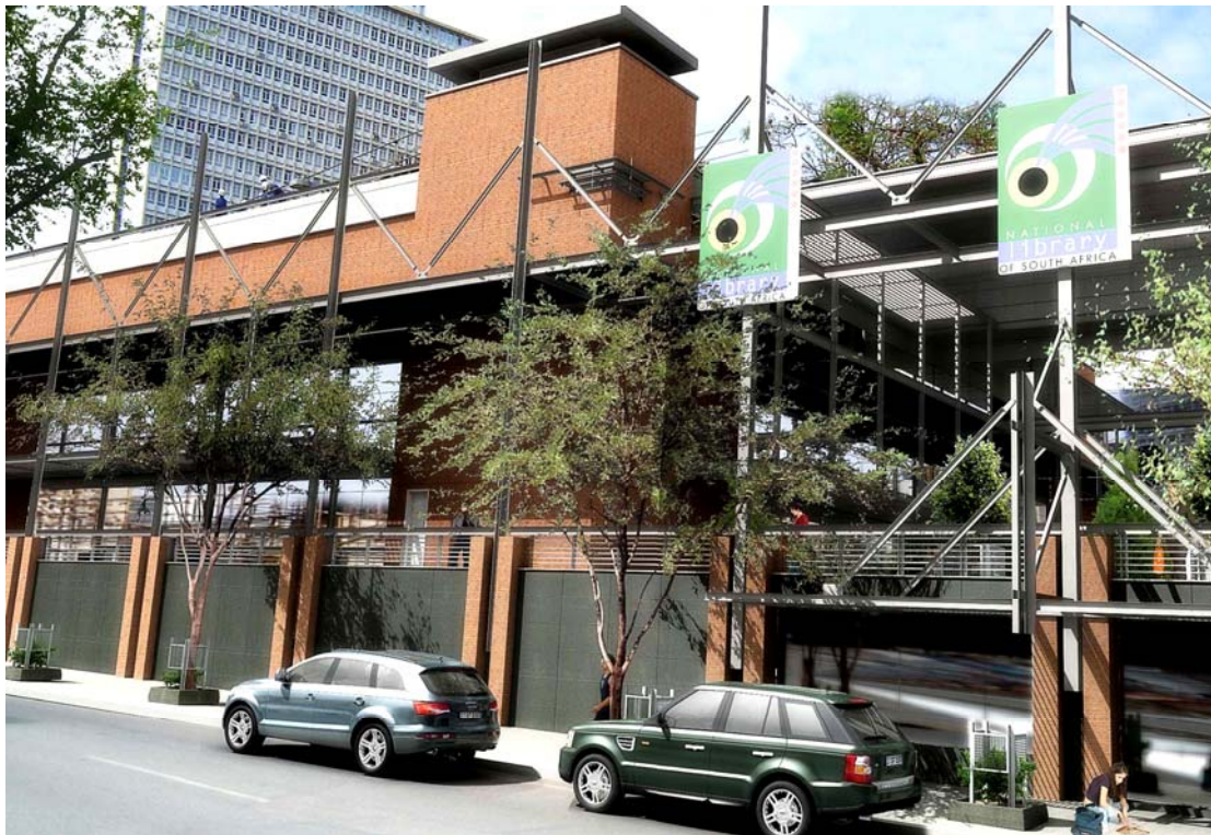
Architect's model of the new building for the National Library of South Africa in Pretoria. (Courtesy of the NLSA and Jeremy Malan Architects and Interiors)
