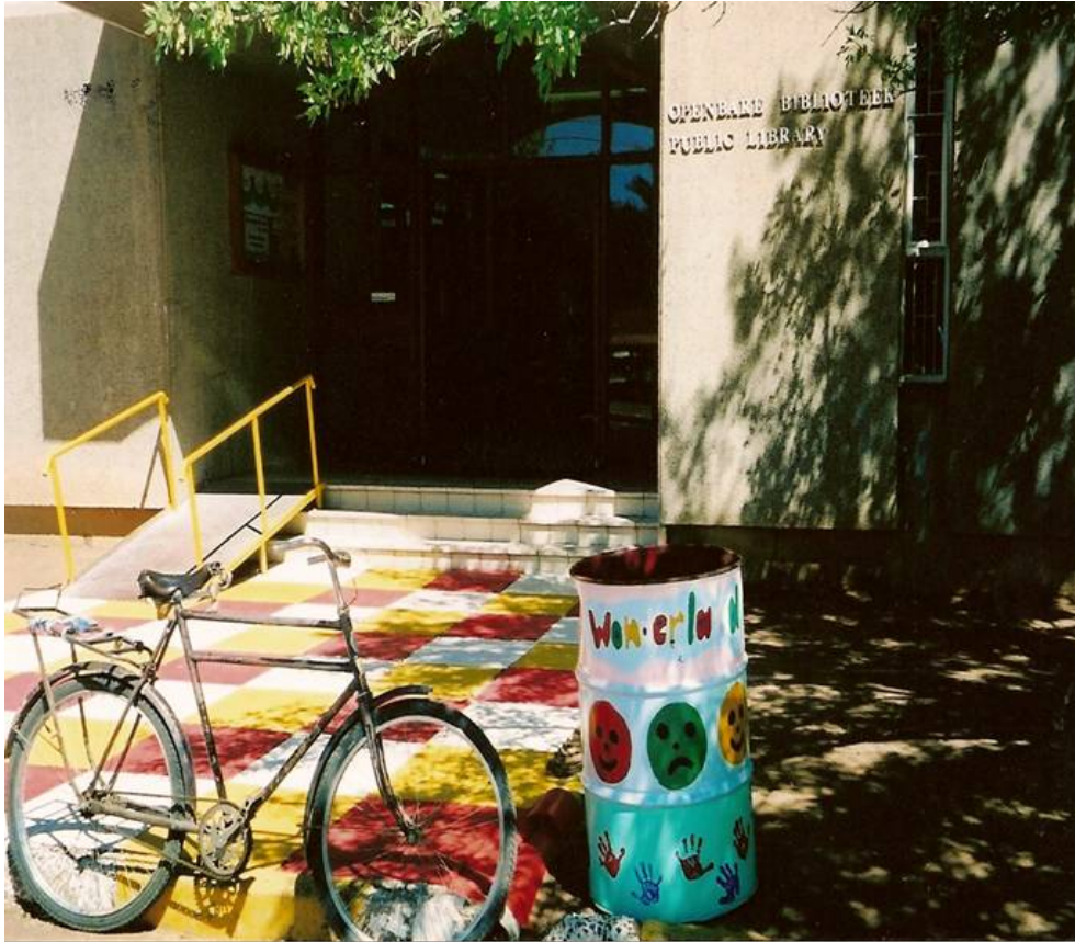
A colourful entrance to the Koffiefontein Public Library in the Free State. The town was originally a diamond mining centre in 1892. (Courtesy of the Directorate of Information Services and Heritage, Free State)
